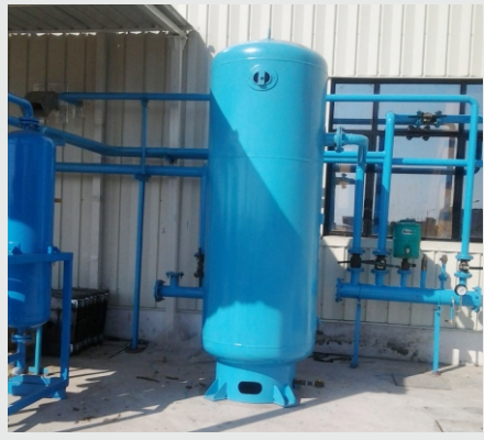
AIR COMPRESSOR PIPE LINE WORK
